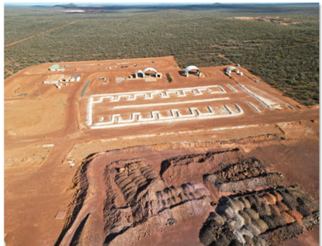
Figure 4: Shine Mine infrastructure
